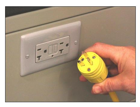
3. Power up the HJ-30i by switching the breaker switch to "ON" (the orange indicator should glow), and pulling out on the Emergency Stop/Power Switch (the red center of the button should glow). Note that only the Power Switch need be pressed in to power down the machine, the other switch can be left in the "ON" state.
